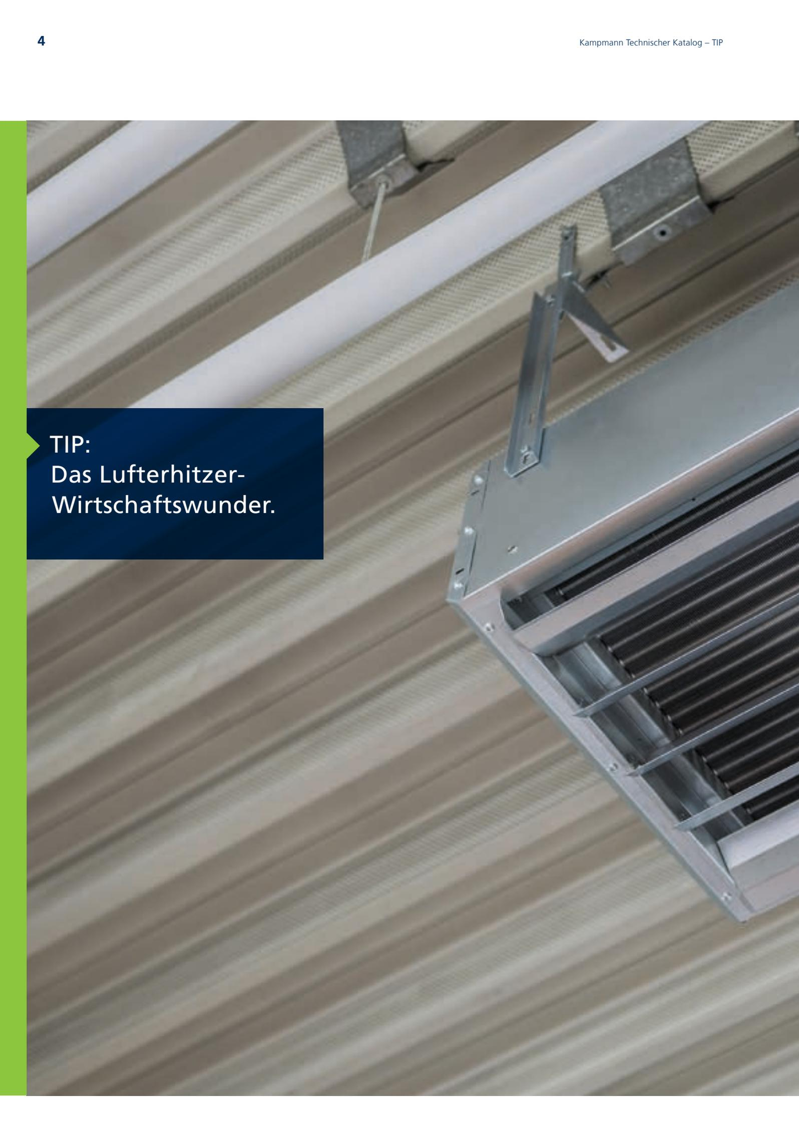
A close-up photograph of a metal air heater unit installed in a ceiling grid. The unit is made of silver-colored metal and features a series of horizontal slats. It is mounted to the ceiling grid using metal brackets and screws. The ceiling grid consists of light-colored, perforated metal panels. The background is a blurred view of the ceiling grid and other similar units.
