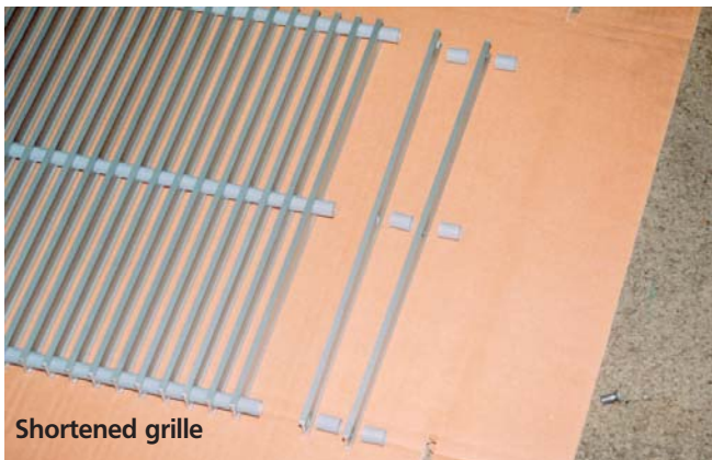
Step 6: Shortening the remaining springs of the grille
