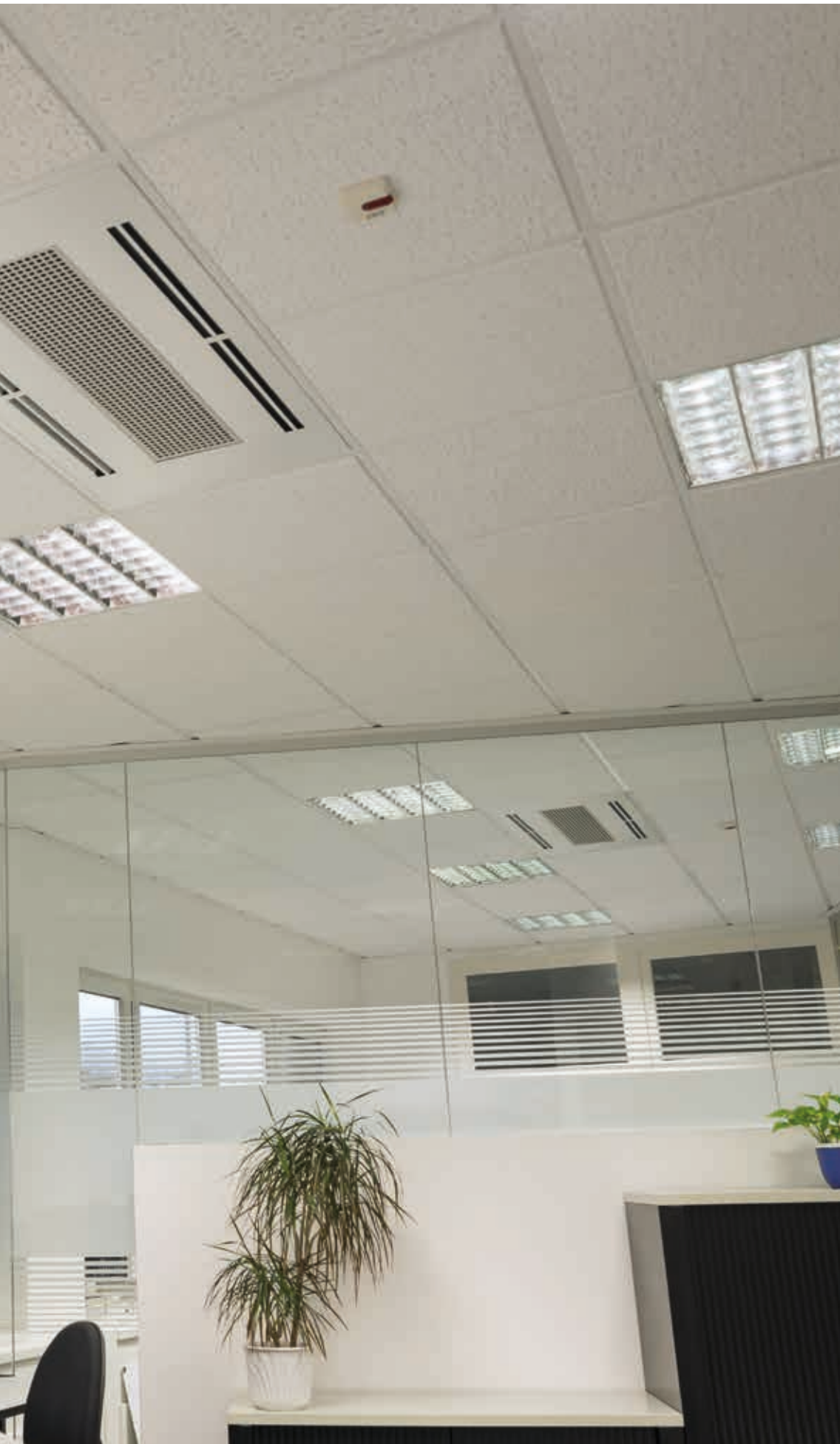
The KaDeck represents a visually discreet room cooling and heating unit. The supply of fresh air is optional.
