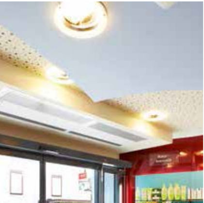
Cassette UniLine Filters can be changed with ease without the need for a tool.
