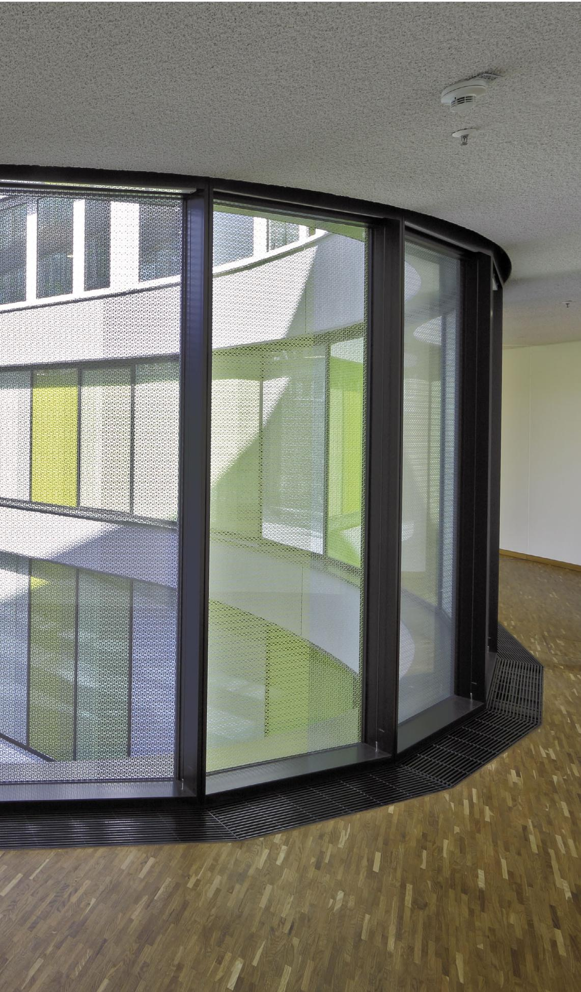
A special design of Katherm HK trench heaters with energy-efficient EC tangential fans ensures quiet operation and energy-savings in the new ADAC head office in Munich (Germany). This design of trench unit produces demand-led filtered, heated or cooled recirculating air from the floor.
